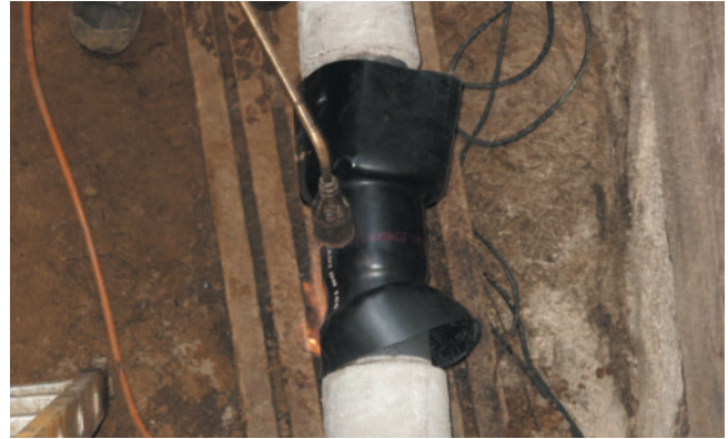
2. Installing the shrink sleeve
