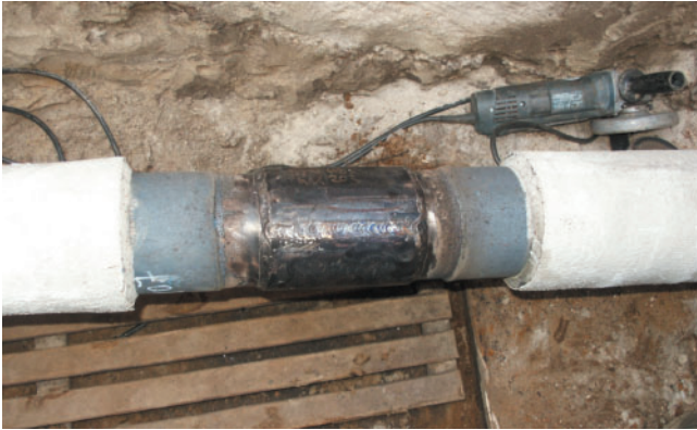
1. Pipe preparation as per GW 15, clean, dry and free of grease. If shrink sleeves are used, preheat to 70°C.
