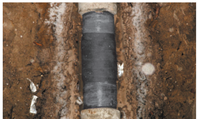
6. Pipecast after application.
