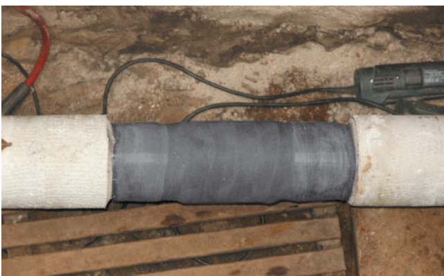
5. Allow the Pipecast to cure for 20-30 minutes at 23°C. It is ready to be buried after in approx. 1 hour.
